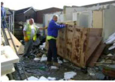
Builders demolishing the old toilet block
